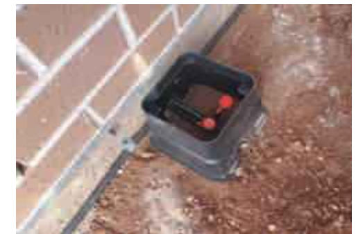
Pic 6 Fit Valve Box
