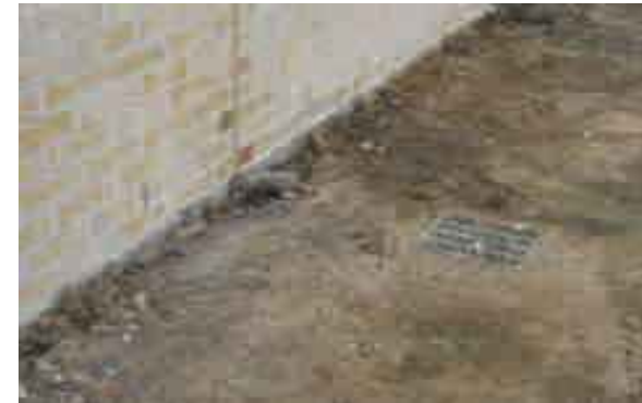
Note drain adjacent to building
