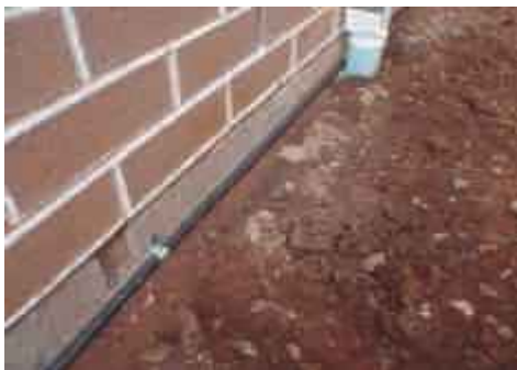
Pic 3 Pipe behind downpipes
