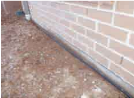
Pic 2 Nail on the clips/pipe
