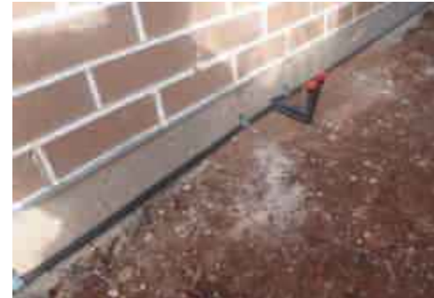
Pic 5 Fit elbows / connectors
